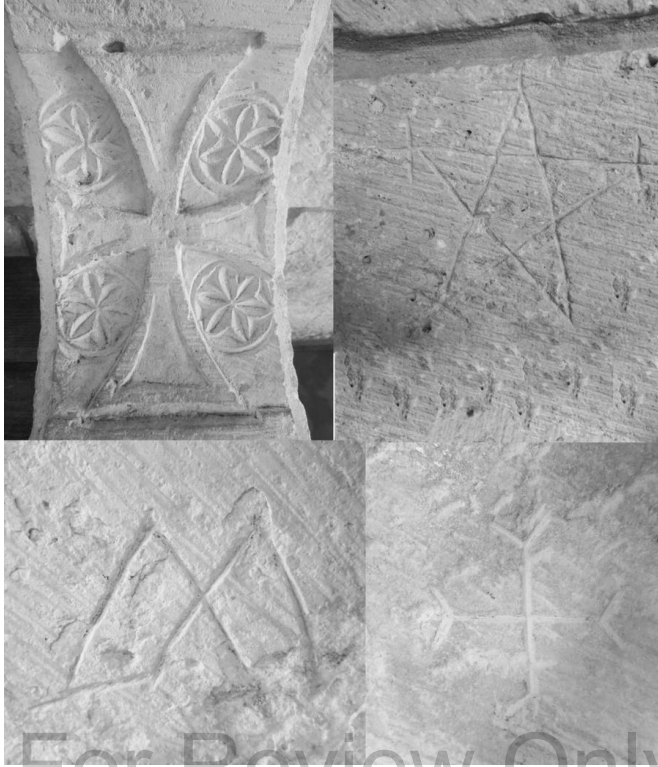
Stone carvings and witch marks of the former St. Bernard of Clairvaux monastery. Clockwise from top left: Cross similar to Cathar and Templar crosses, surrounded by patterns similar to the flower of life design; pentagram; stylized cross; and MM sign.
